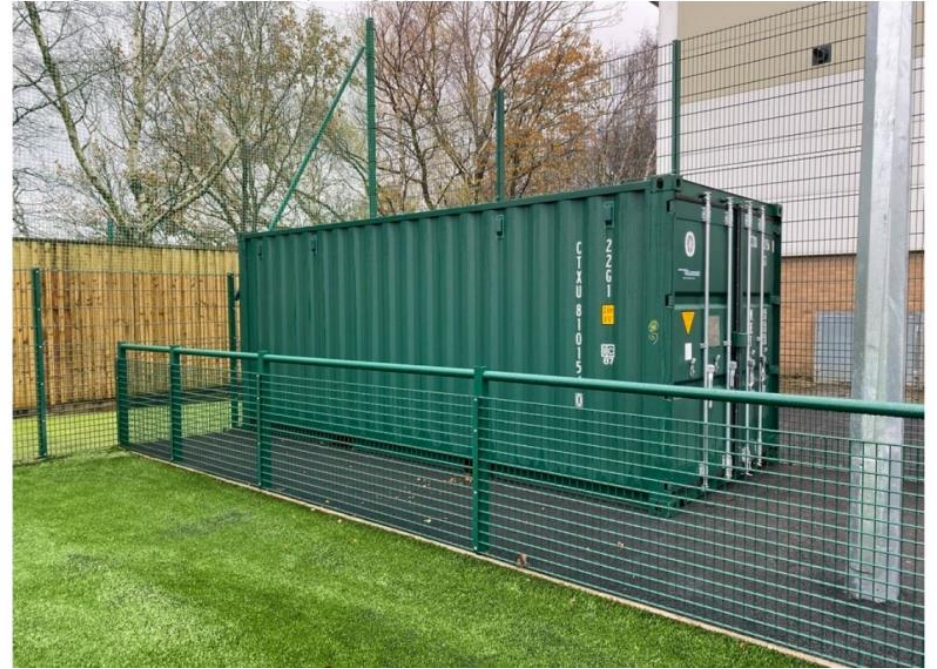
1.2m high Twin Bar Super Rebound spectator rail:
